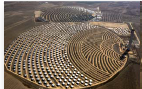
Picture 2: PS-20 built by Abengoa (Source: RENAC, 2010)
